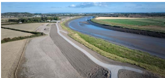
Pawlett primary embankment
