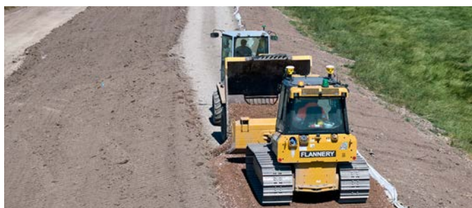
Crew applying stone on the crest of the primary embankment near Combwich, which will form part of the public right of way
