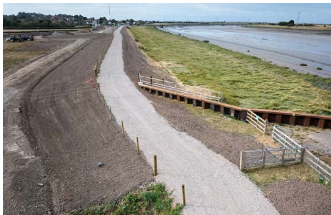
Tucketts Clyce outfall structure and the primary embankment near Combwich
