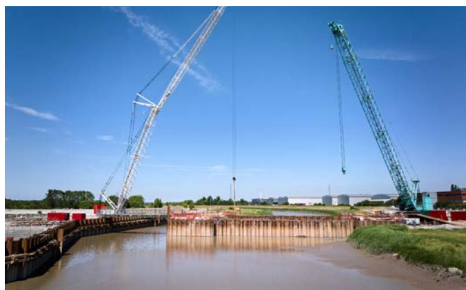
Looking downstream with cofferdams being accessed by crane
