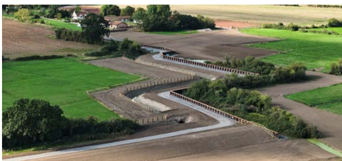
Seepage cutoff wall at Perry Wood
