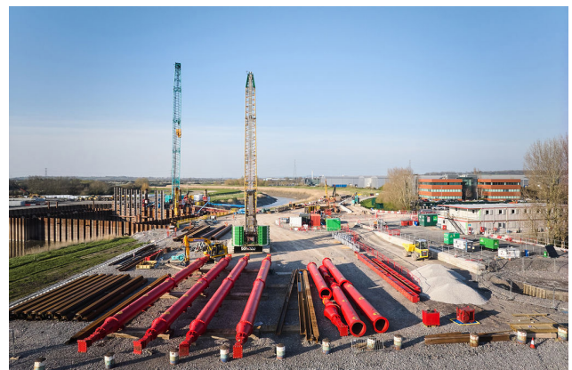
Propping on site and ready for installation
