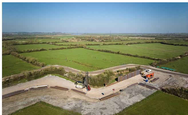
Seepage cut off wall piling installation has begun
