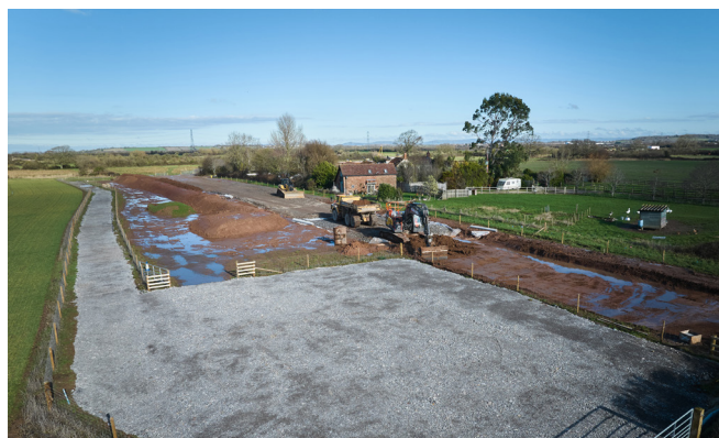
Piling mat installation
