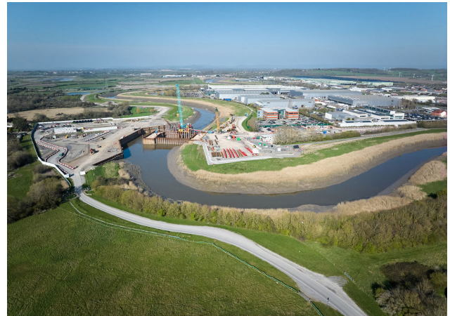
Birds eye view of the barrier substructure
