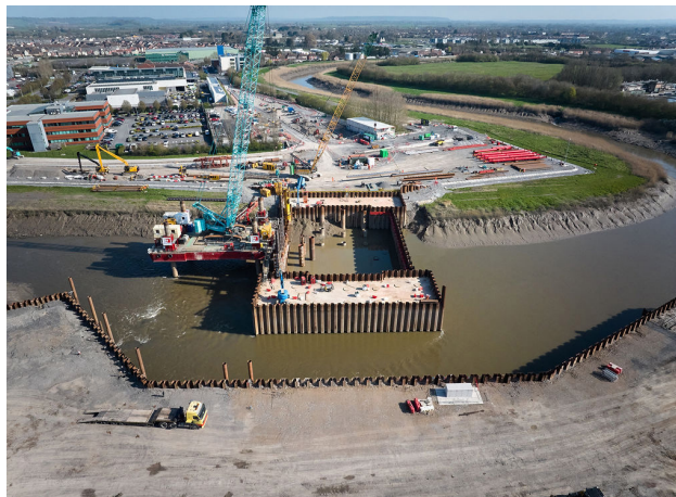
Bypass channel is now complete and in use
