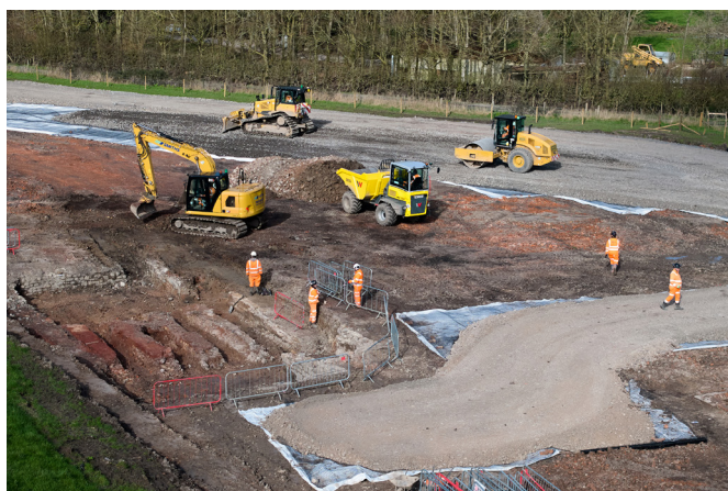
Continuation of the haul road construction
