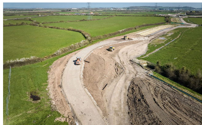
Continuation of the secondary embankment
