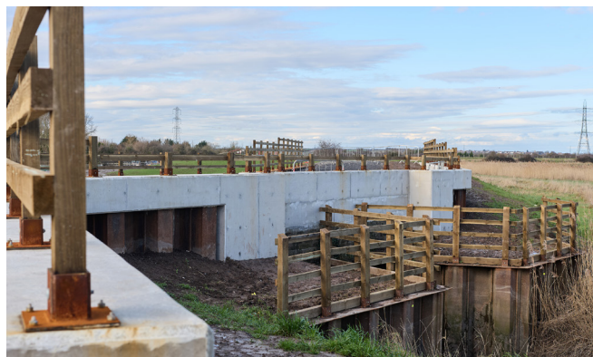
Pims Clyse Outfall Structure concrete capping beam
