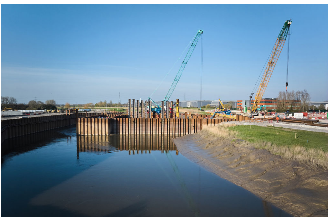
Southern central cofferdam sheet pile wall is complete
