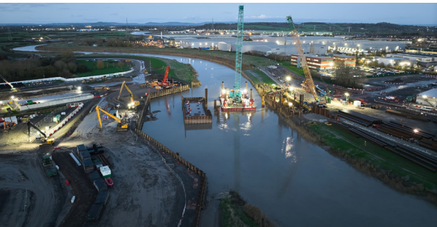
Aerial view of the temporary bypass channel at high tide
