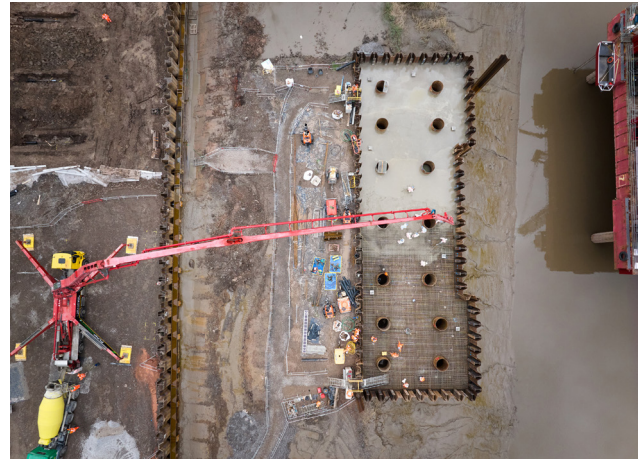
First concrete pour for the temporary tension slab in the west cofferdam
