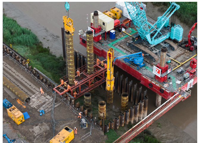
Tubular piles – West cofferdam
