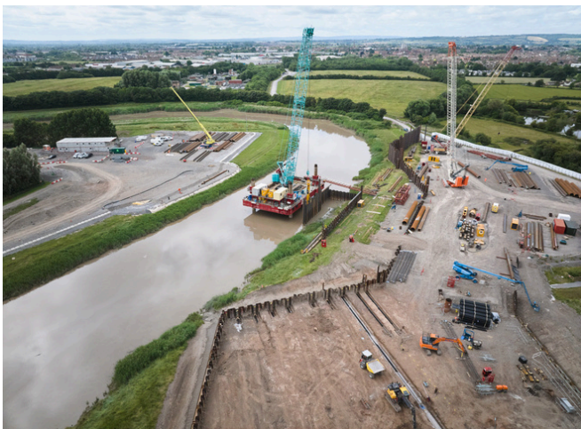
Bypass channel piling
