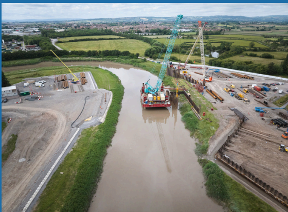
Load Transfer Platform (Left hand side)
