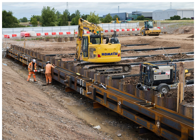
Anchor wall installation
