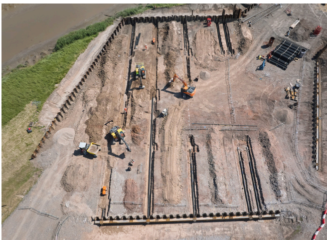
Tie rods installation
